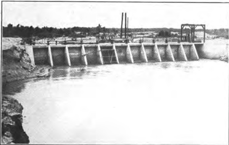
The Cement Intake Gate Came After the Valley Was Well Advanced in Reclamation
