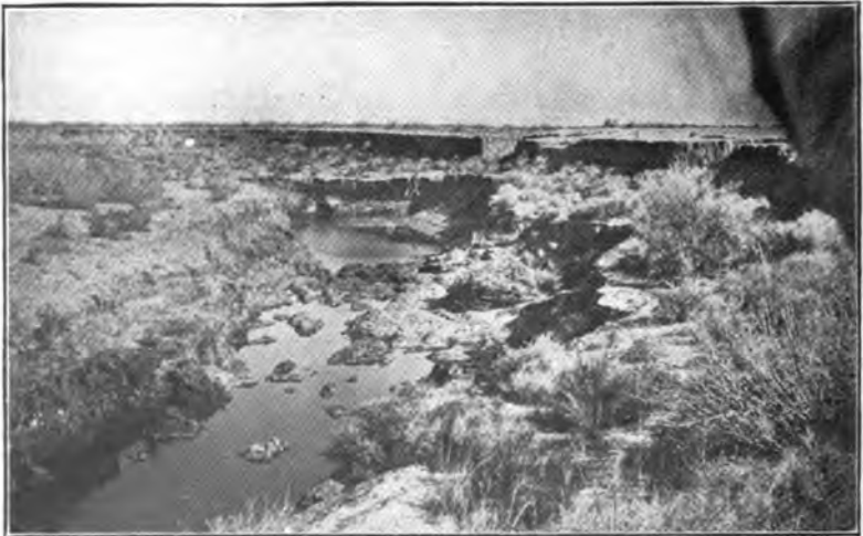
Before the Canal was Built to Imperial Water was Hauled from a Sink in New River
