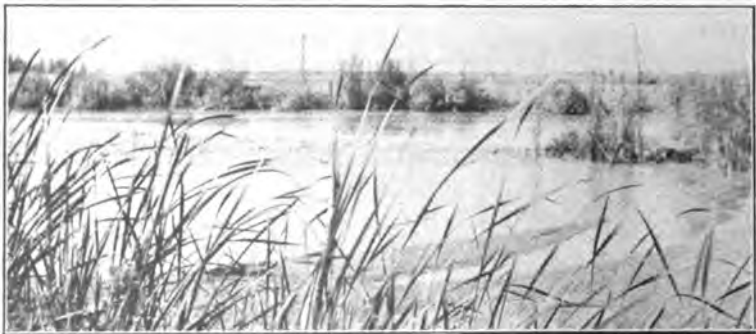
Graphic Illustration of Land Building by the Waters of the Colorado is Found in Some of the Ditches. In this Case the Two Mud Dams Shown in the Foreground Were Built Up in a Channel Eight Feet Deep and Rose Above Water Surface in Four Months.
