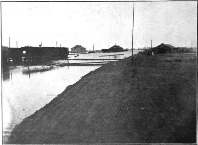
The Town of Calexico was Protected by a Dike
