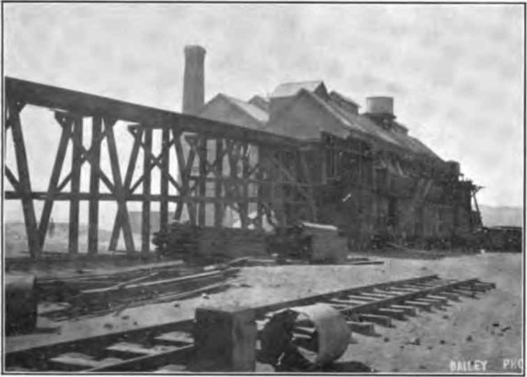
BORAX WORKS, SAN BERNARDINO COUNTY.
