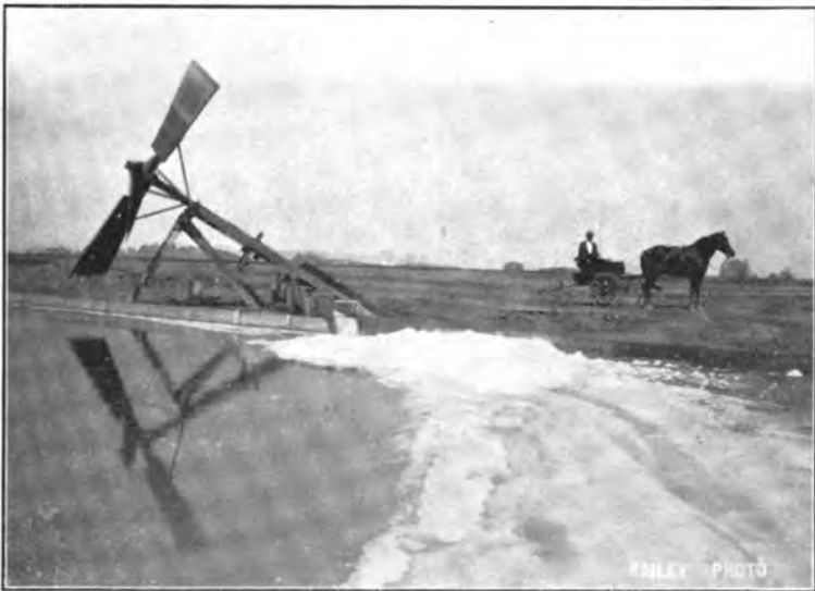
ARCHIMEDES SCREW WINDMILL—ALAMEDA SALT WORKS. USED FOR PUMPING BRINE FROM THE TANKS.
