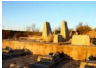
Remains at the Brunckow Mine.
