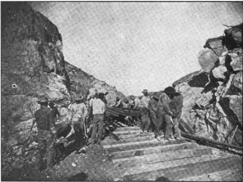
WORK LIKE THIS IS GOING ON AT MANY POINTS IN ARIZONA
