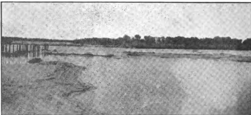
LOOKING SOUTH ACROSS INTAKE NO. 3, JULY 18, 1905. THE REMAINS OF SECOND ATTEMPT ARE VISIBLE
