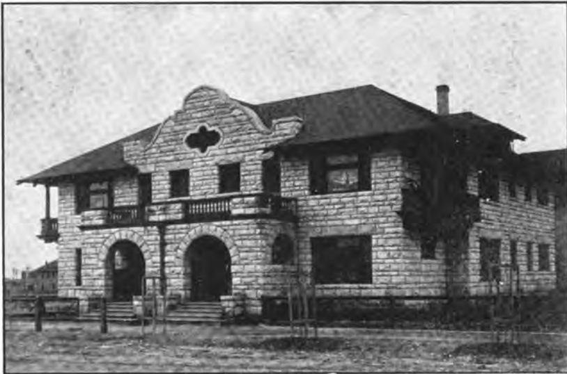
▲ RESIDENCE AT DOUGLAS
