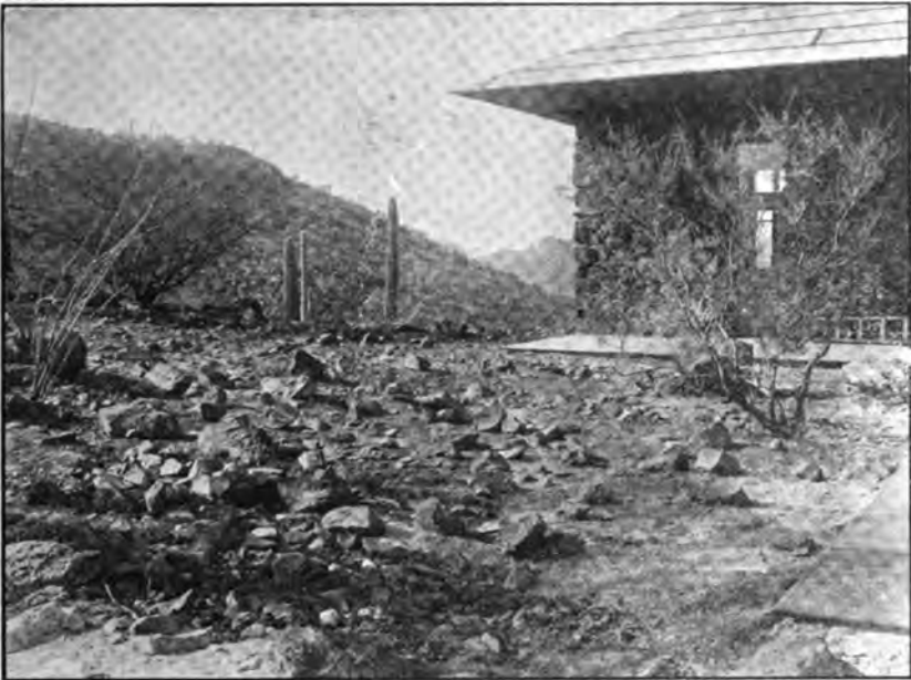
A CORNER OF THE LABORATORY, LOOKING SOUTHWEST
