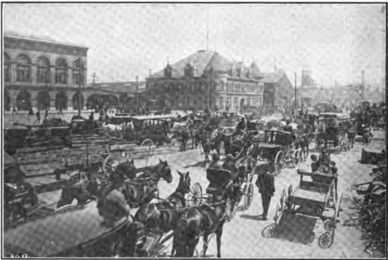
EAST STREET SOUTH FROM MARKET SHOWING FERRY POST OFFICE Photograph taken May 10, 1906
