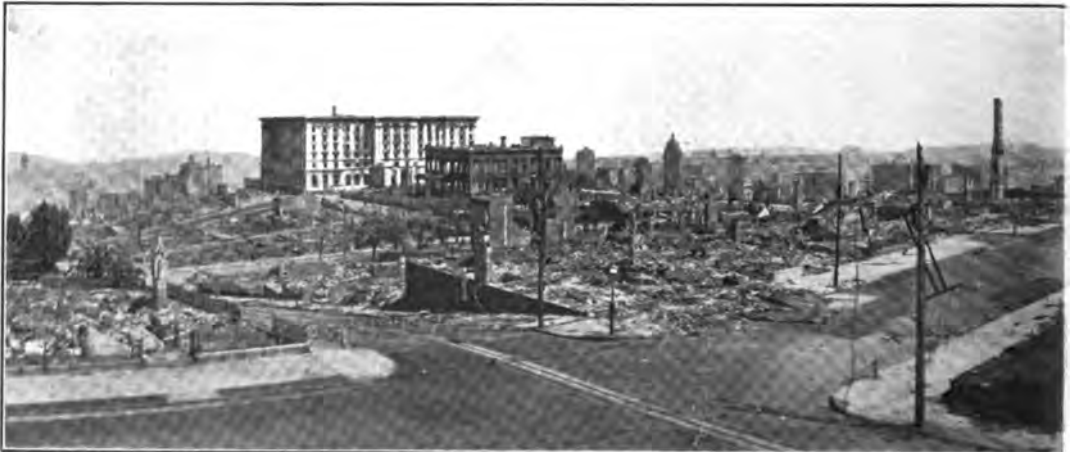
LOOKING SOUTH FROM CORNER
