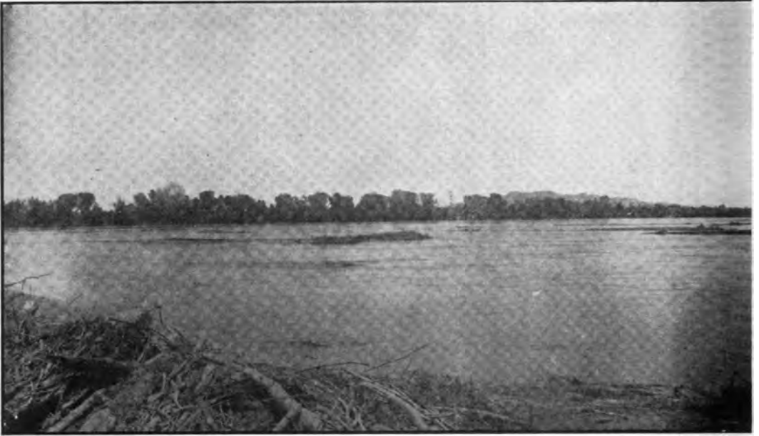
VIEW FROM ISLAND IN RIVER, LOOKING NORTH
