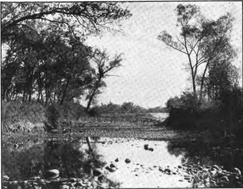
Intake to Main Canal from New Weir, Kings River, at Low Water.
