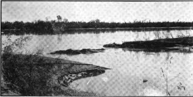
INTAKE NO. 1 FROM NORTH BANK, JAN. 22, 1905
