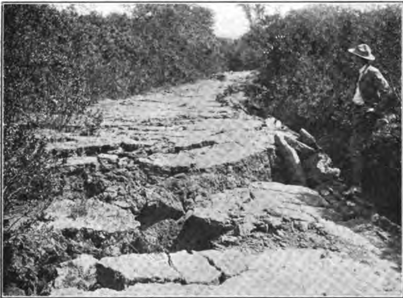
BREAK ALONG THE STEVENS CREEK FAULT Five miles southeast of Stanford University
