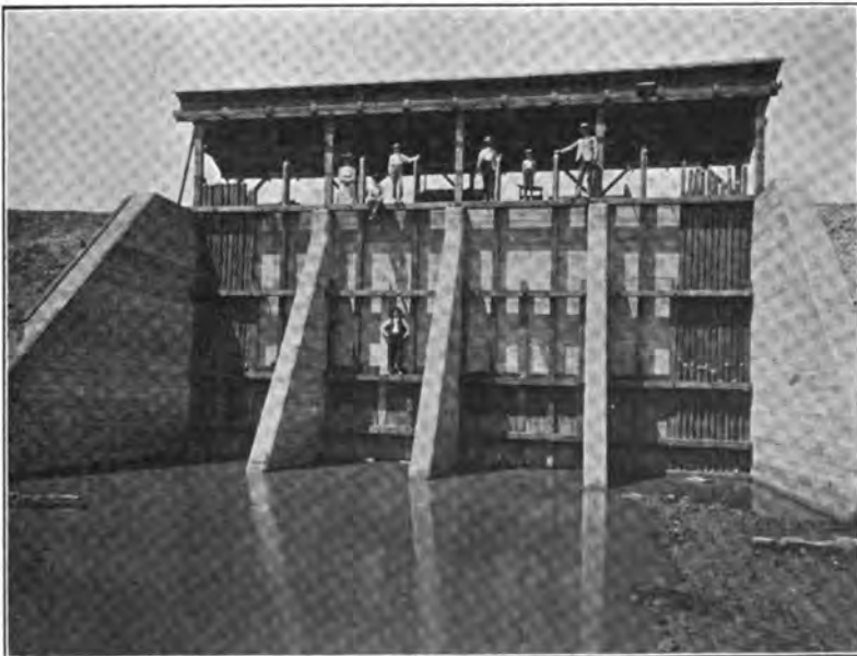
Head Gate Butte County Canal
