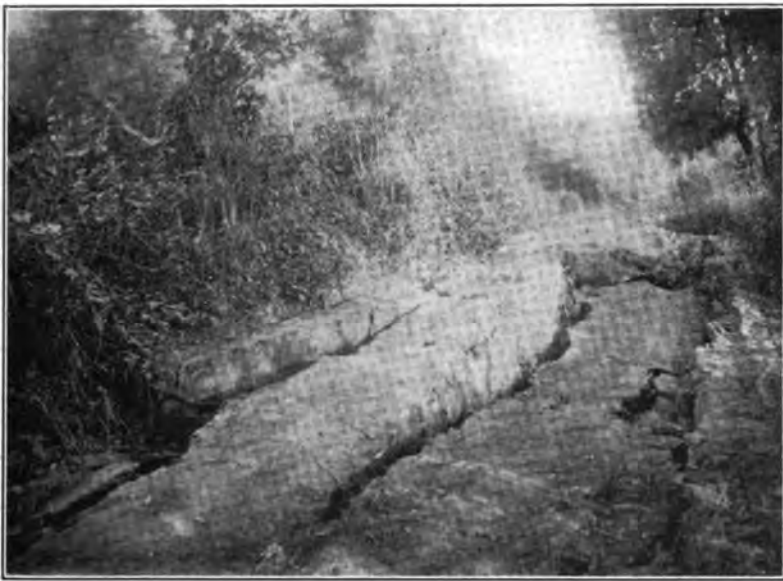
FRACTURE IN A ROAD BETWEEN MILPITAS AND ALVISO, SANTA CLARA COUNTY
