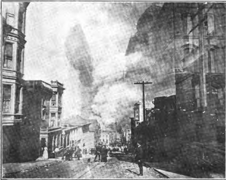
LOOKING EAST ON SACRAMENTO STREET DURING FIRE
