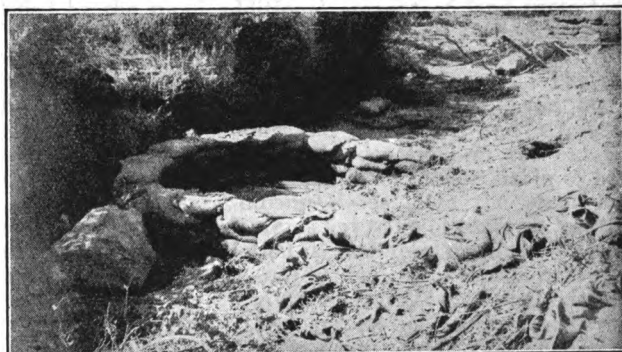
FIG. 76.—SAND "BOILS" HOOPED WITH SAND SACKS.
