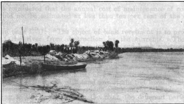
FIG. 80.—LEVEE PROTECTED BY ROCK.
