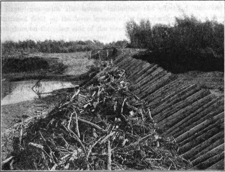
FIG. 10.—TYPICAL ABATIS WORK ON LEVEES OF YUMA PROJECT, U. S. RECLAMATION SERVICE.
