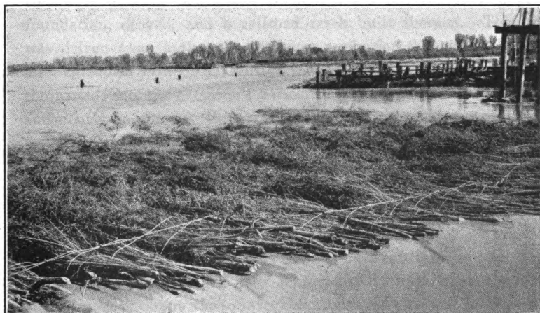
FIG. 31.—DOWN-STREAM END OF BRUSH MATTRESS ABOVE WATER BECAUSE OF SILTING ACTION.
