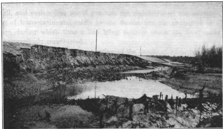
FIG. 41.—EFFECT OF FLOOD OF DECEMBER 7TH, 1906, ON LEVEE OF U. S. RECLAMATION SERVICE, OPPOSITE LOWER HEADING.
