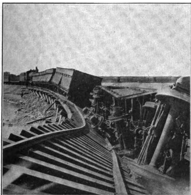
The First Load on the Trestle Caused a Wreck
