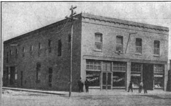
New Thing Building, Calexico
