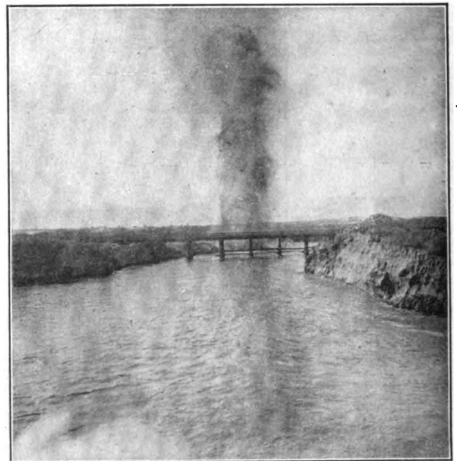
Blasting in the Main Channel
