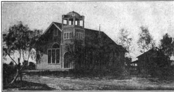
New M. E. Church, Brawley
