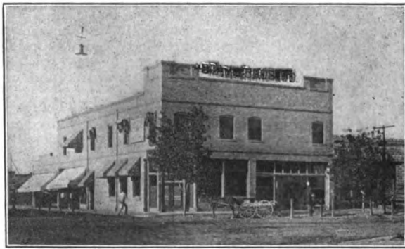
Imperial Valley Bank Building
