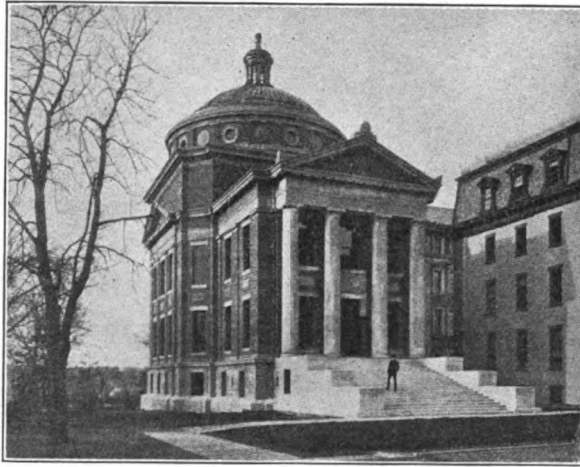
EARL HALL, COLUMBIA UNIVERSITY. This building is the headquarters of the American Association and the affiliated societies.
