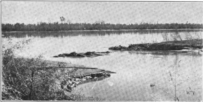
INTAKE No. 1, from North Bank. January 22, 1905.
