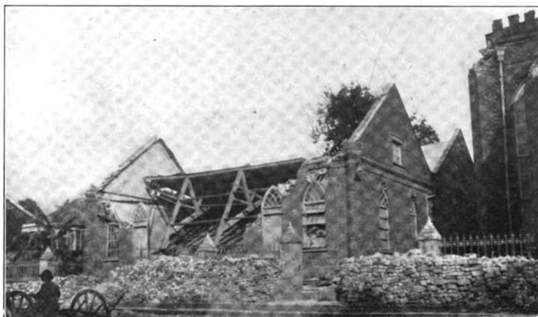
FIG. 8, b. EAST AND WEST WALLS CRUSHED.
