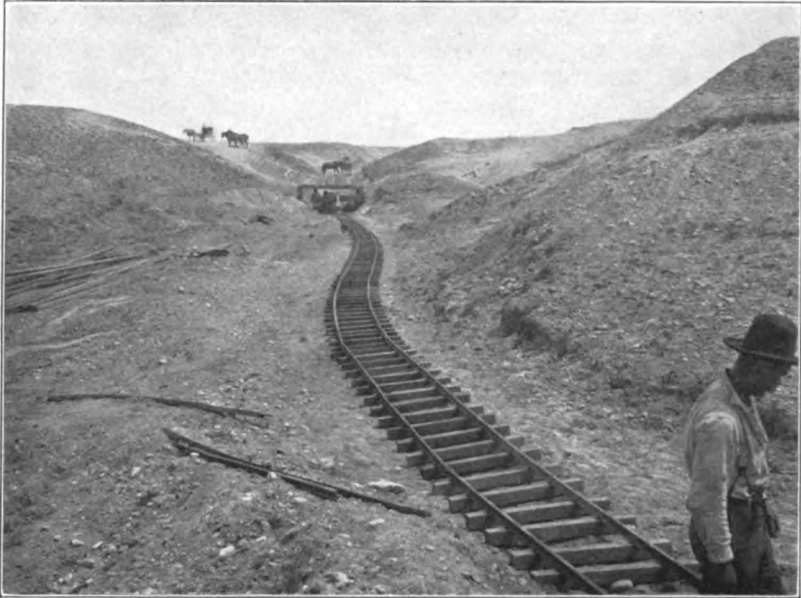
FIFTY-FOOT CUT ON THE INTERSTATE CANAL.
