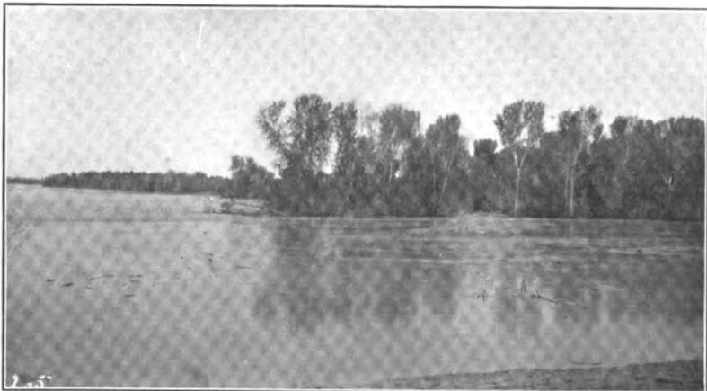
VIEW LOOKING SOUTH ACROSS INTAKE No. 3. May 29, 1905.
