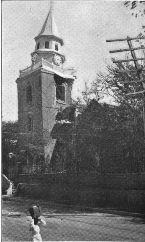
FIG. 3. TOWER OF PARISH CHURCH SHATTERED AND INCLINED TO THE EAST. Stopping of clock by shock.
