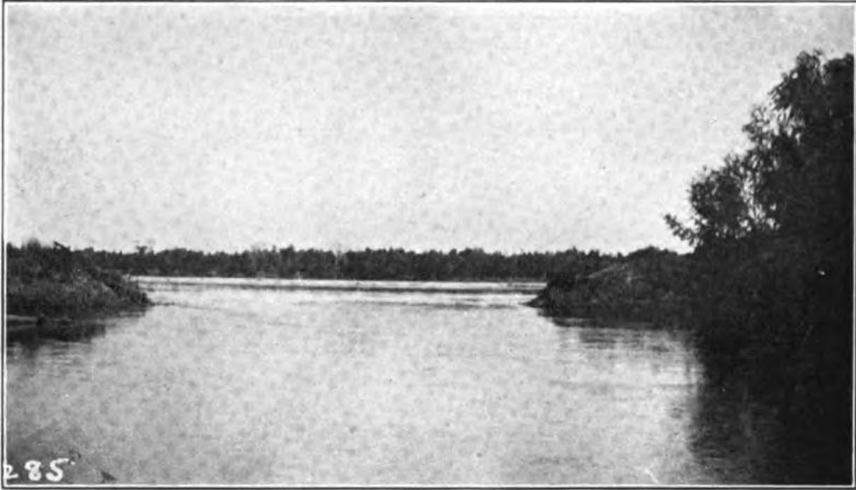
INTAKE No. 2, looking out toward the river. October 17, 1905.
