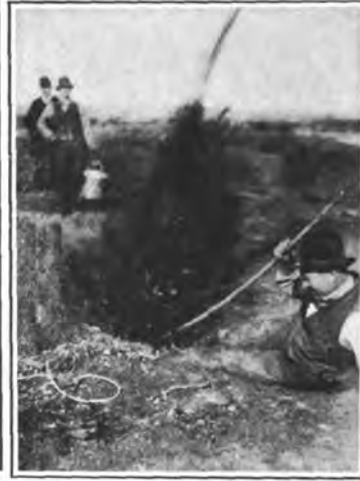
BLOWING OUT A HOLE FOR THE STUMP-LIFTING CHARGE.
