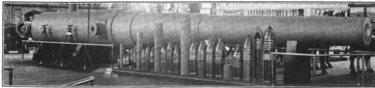
THE MOST STRIKING FEATURE OF THE WAR DEPARTMENT EXHIBIT. Full sized model of a sixteen-inch coast-defense rifle, the largest ever made, weighing 141 tons and throwing a projectile weighing 2,400 pounds a distance of twenty-two miles.
