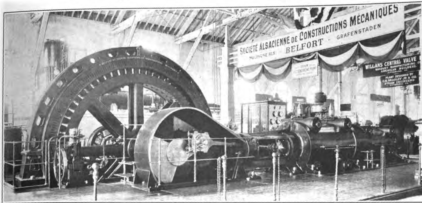
700 KILOWATT, THREE-PHASE ALTERNATING CURRENT GENERATING SET.
