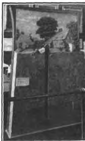
WATER INFECTION. Model showing how wells are polluted.
